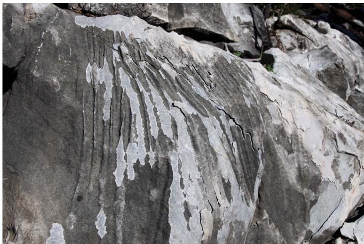
Figure 1 (above) Rillenkarren damage in the West Deep Creek area caused by the January 2020 bushfire.
